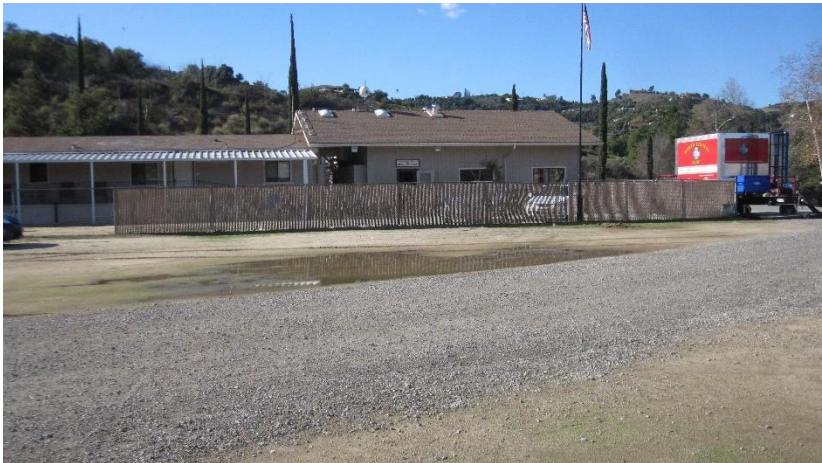
Photograph 1. View of the onsite fire station building, facing east.
