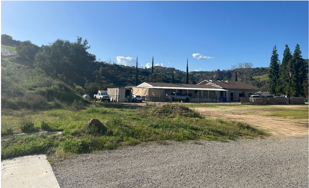
Photograph 1. View looking northwest from the eastern project boundary showing existing fire station. March 2024.
